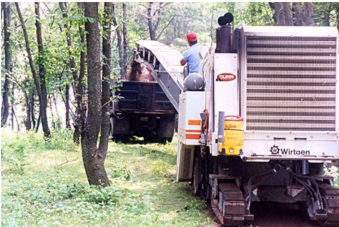
Forsyth Bike Trail Construction
