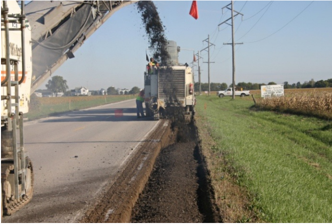
Surface removal/trench widening
