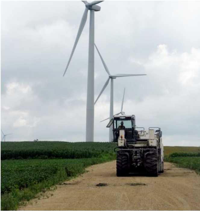
Dekalb County Wind Farm. Pavement Pulverization
