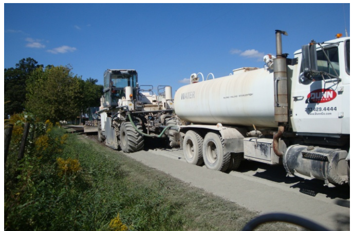
Full Depth Recycling with cement in Rochester township 2010
